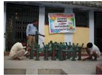
Installation of Handpumps in the village of Madhepura, Bihar
